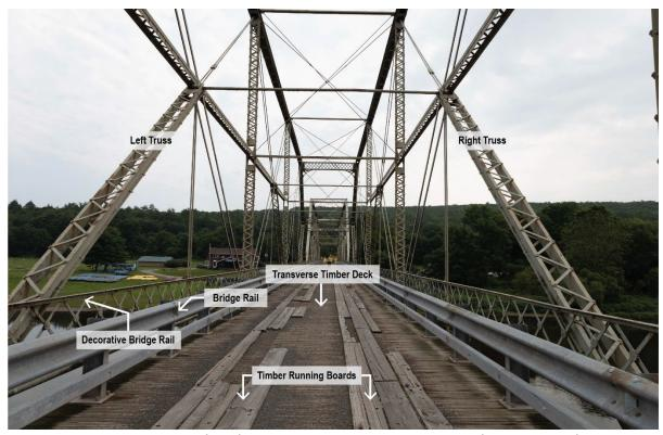
Figure 7: General Bridge Components, Section View Looking Eastward
