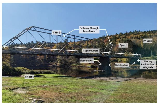
Figure 6: General Bridge Components, Elevation View
